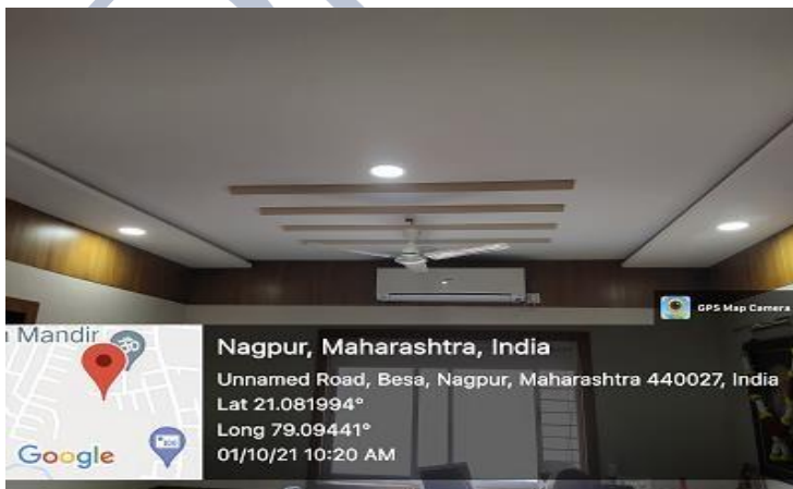
Use of false ceiling to reduce air-conditioned volume and reducing AC load
